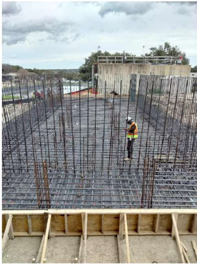
2024.02.16, Rebar Installation for Headworks/Aeration
