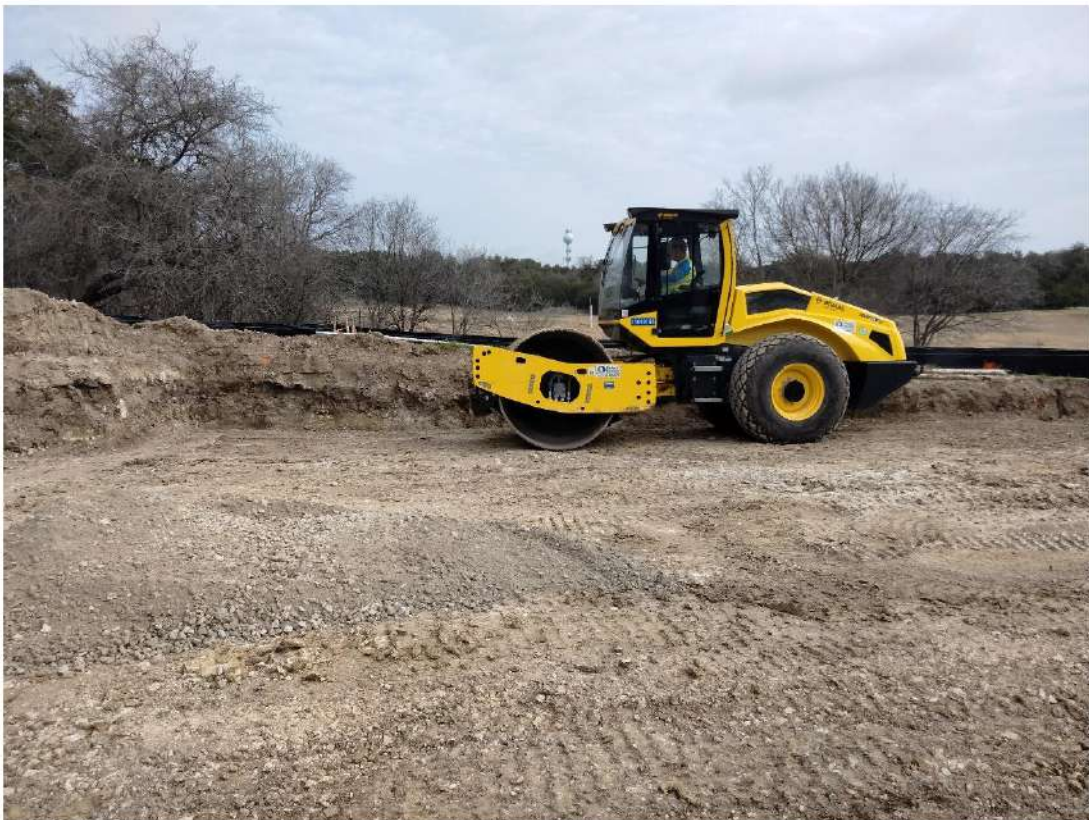
2024.02.08, Proof-rolling Headworks/Aeration Subgrade
