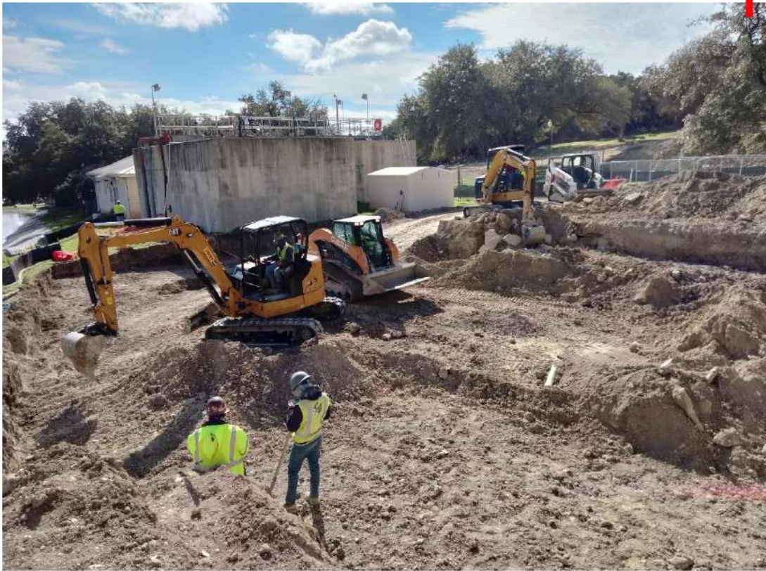
2024.02.07, Excavation for Headworks/Aeration
