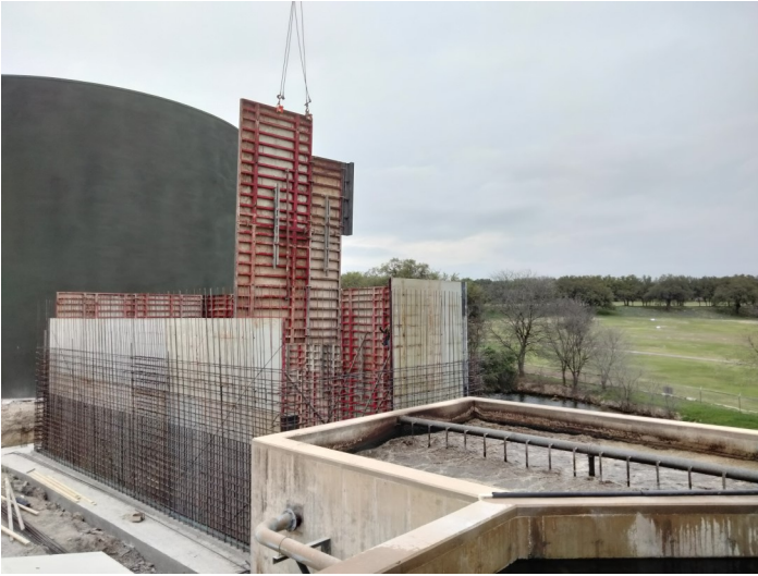
2024.03.07, Aeration Basin Wall Formwork Installation
