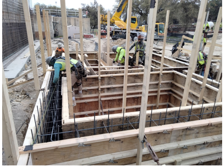
2024.03.07, CL2/Effluent Basin Rebar/Formwork Installation
