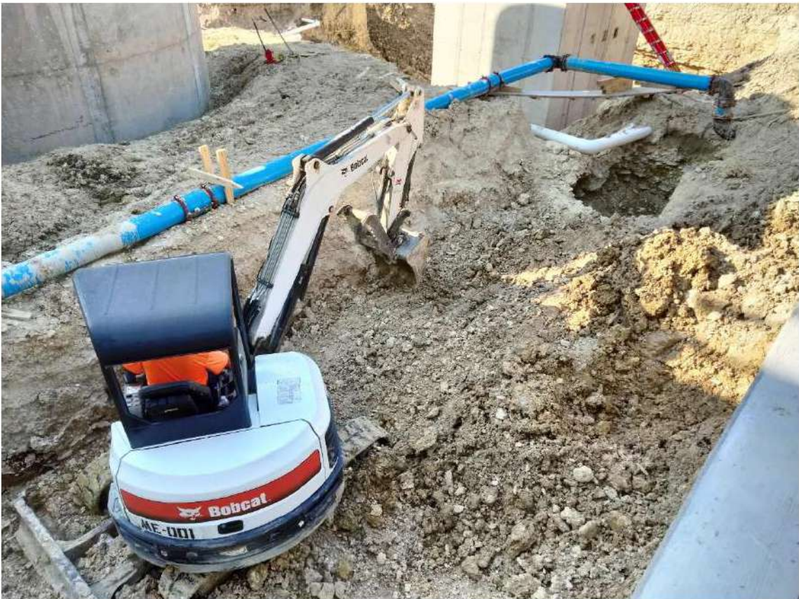
2024.08.06, Excavating for Manholes A2 & C1
