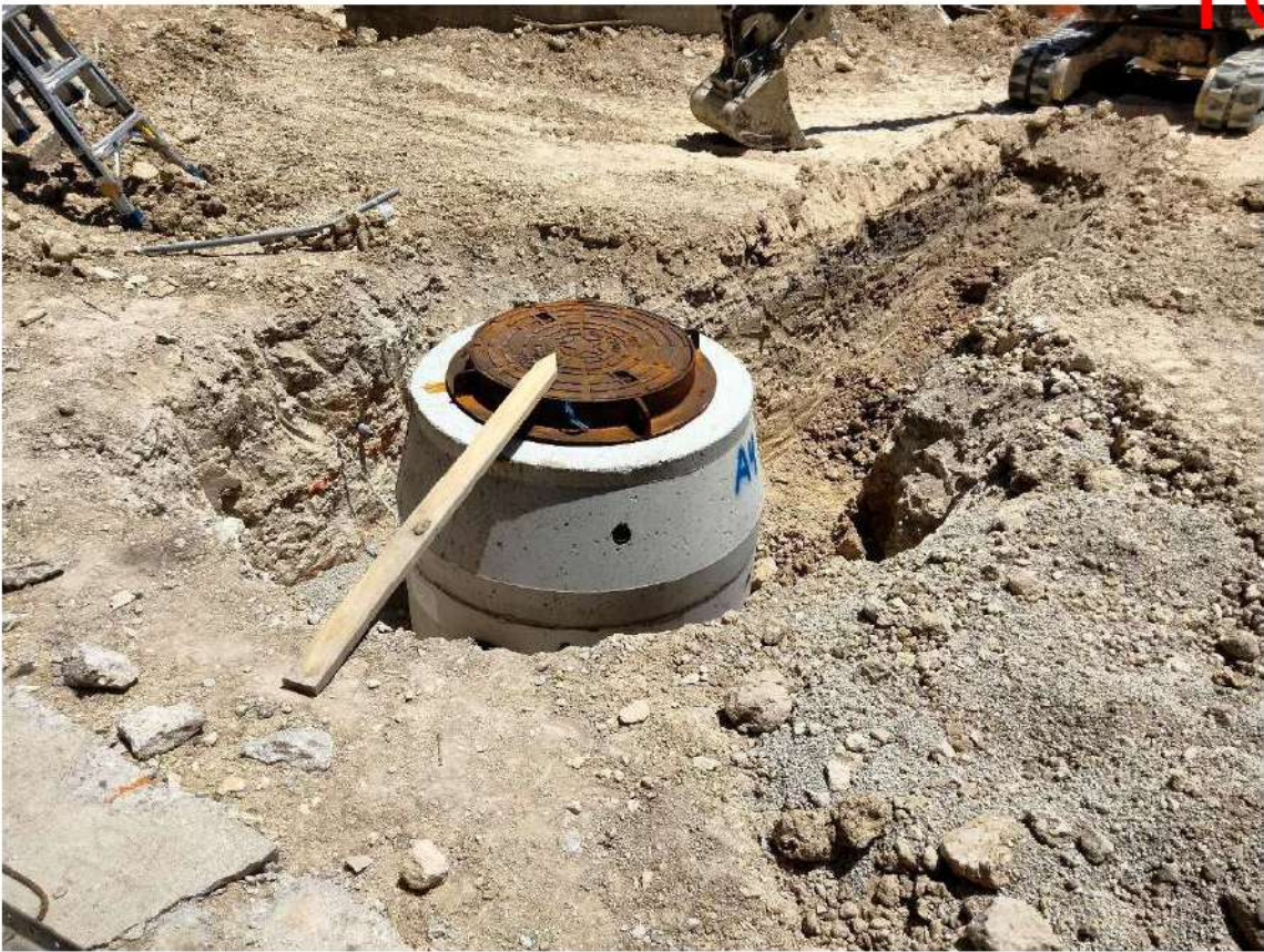
2024.08.13, Installation of Manhole A4
