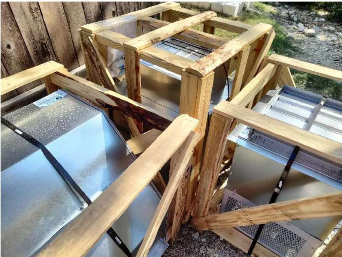
2024.08.12, Delivery of HVAC Equipment
