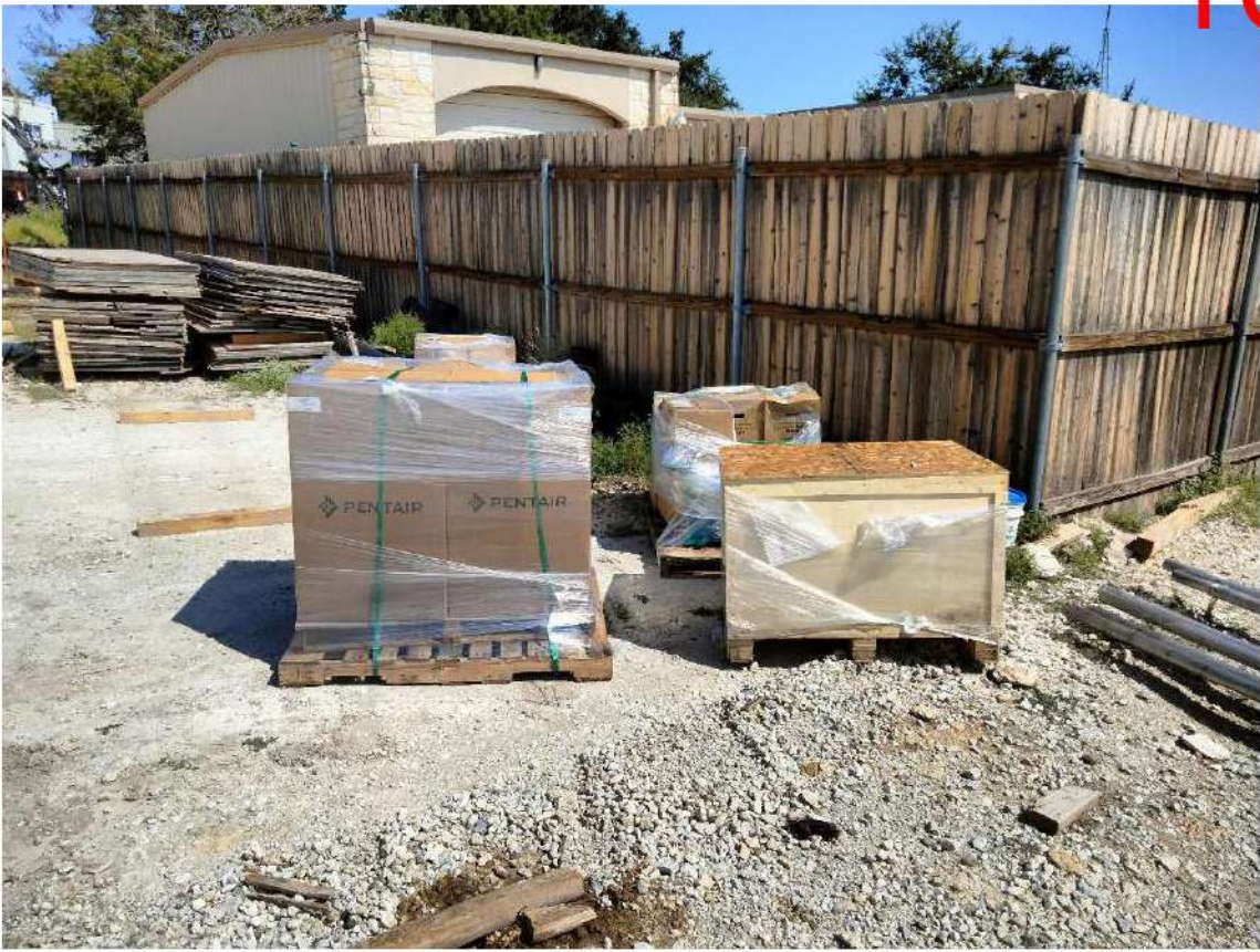
2024.08.06, Delivery of Submersible Pumps & Accessories
