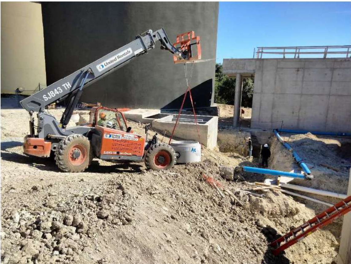
2024.08.19, Installing Manhole A2
