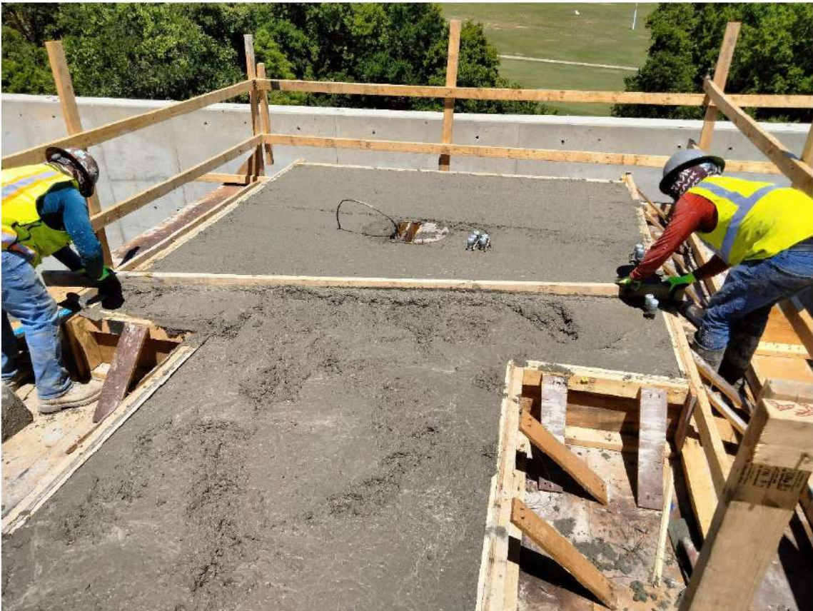
2024.04.11, Screeding East Aerator Platform
