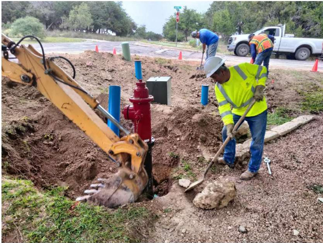
2024.04.16, Backfilling & Re-Grading
