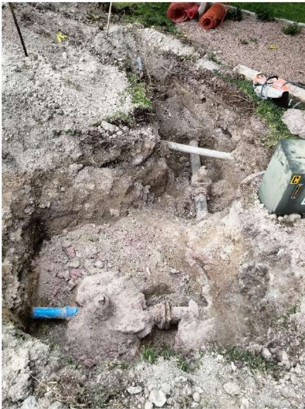
2024.04.15, Exposed Existing Gate Valves & Hydrant at Lakeland Dr / Lakepoint Cir
