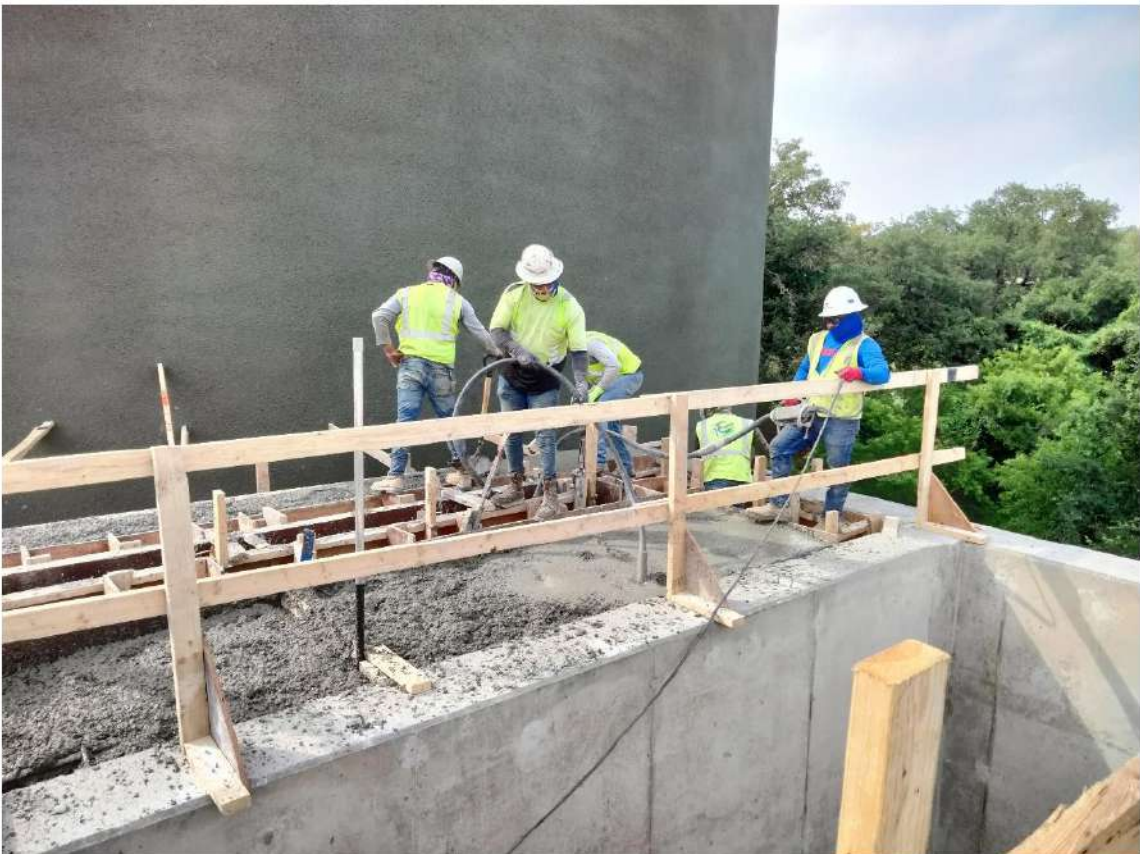
2024.04.18, Vibrating and Screeding Headworks Channels and Top Slab
