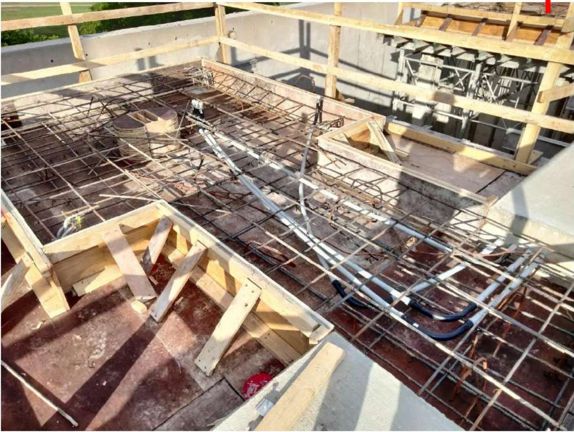
2024.04.10, West Aerator Platform Formwork & Rebar Installation
