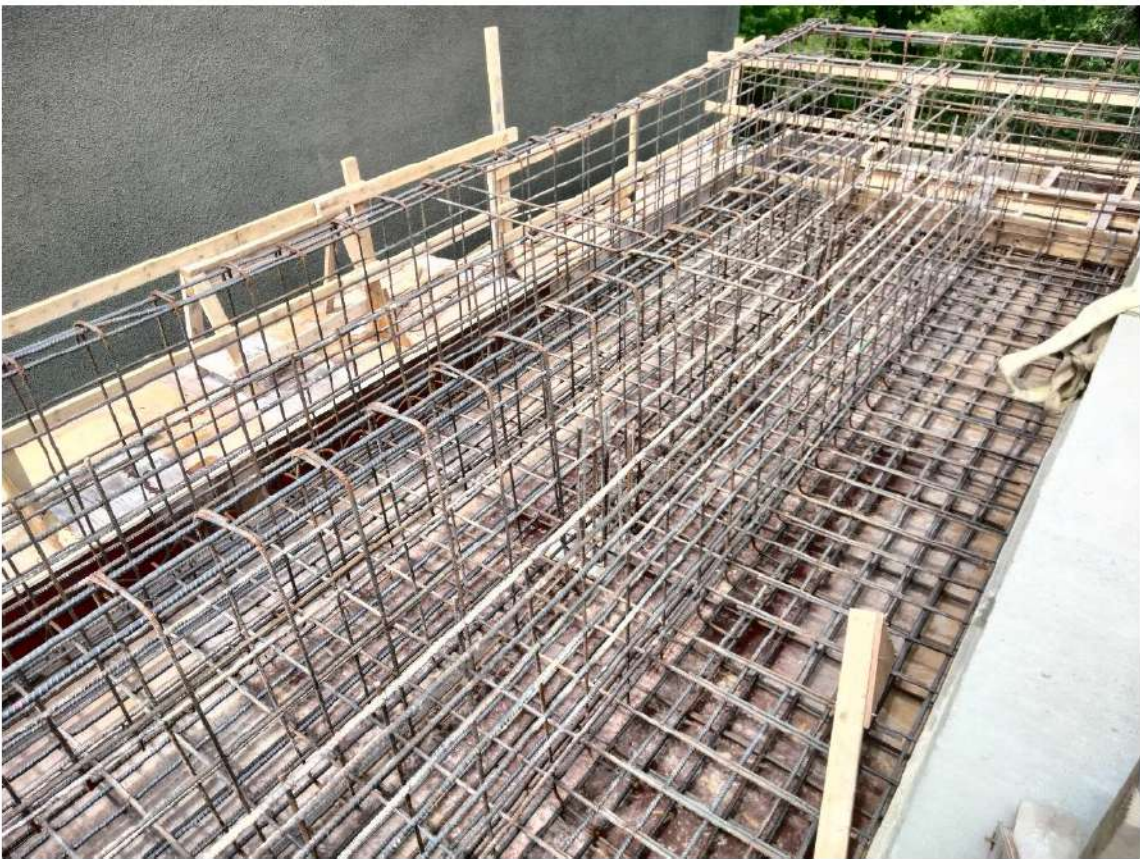
2024.04.10, Headworks Slab Formwork & Rebar Installation
