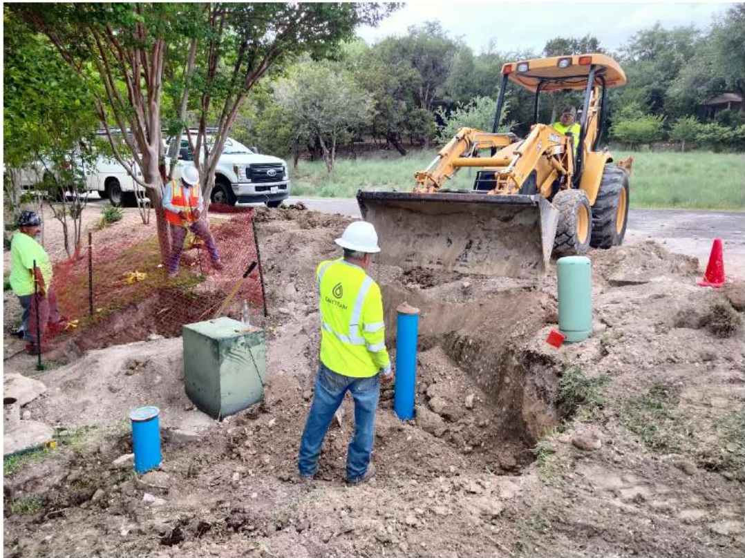
2024.04.15, Backfilling New Gate Valves
