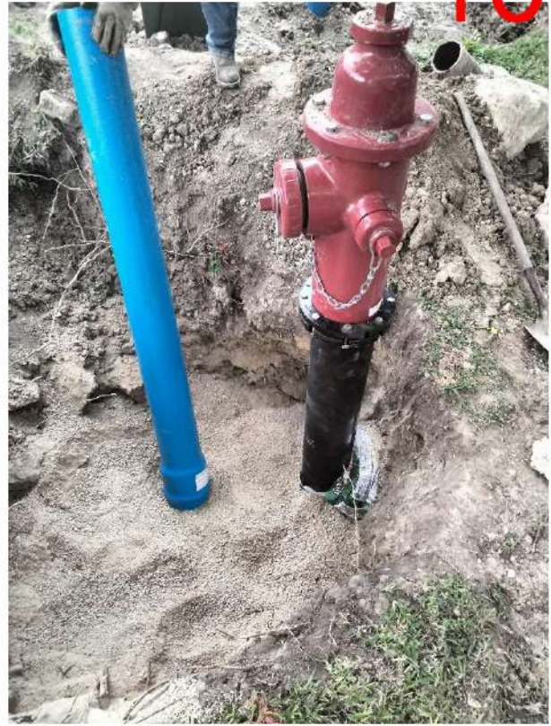
2024.04.16, Pipe Bedding Installation
