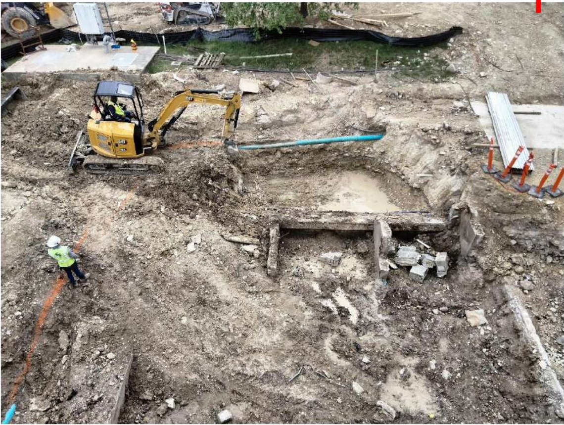
2024.04.10, Excavation for Clarifier
