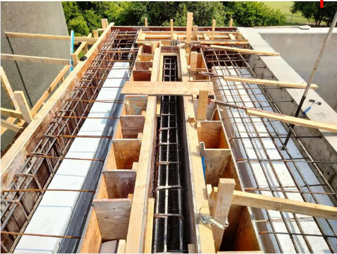
2024.04.18, Headworks Channels and Top Slab Formwork & Rebar
