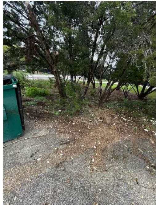
2024.03.22, WTP-Generator Project Site (After)
