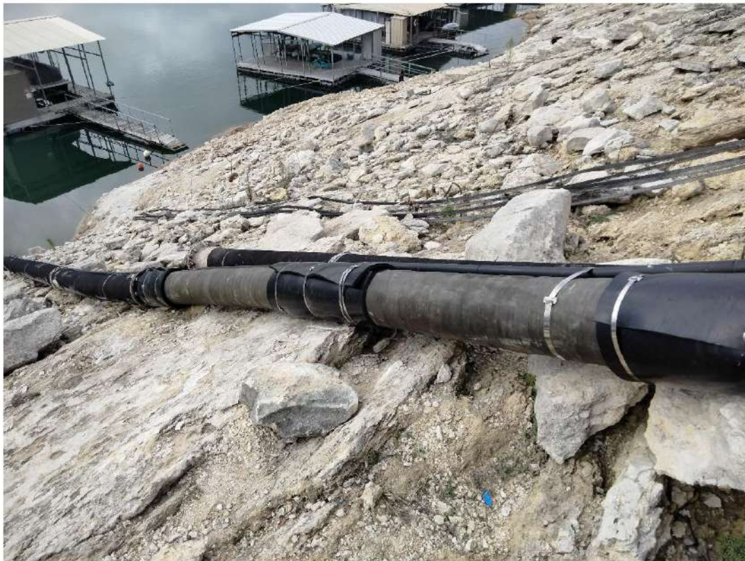
2024.03.04, Installation of Raw Water Hose near Shore
