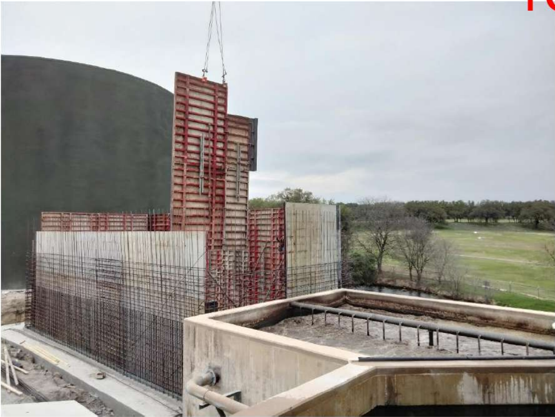
2024.03.07, Aeration Basin Wall Formwork Installation
