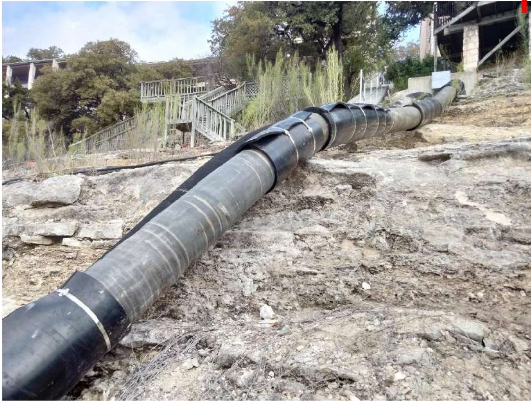
2024.03.04, Installation of Raw Water Hose near Bulkhead Structure
