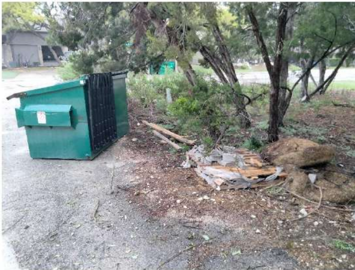
2024.03.22, WTP-Generator Project Site (Before)
