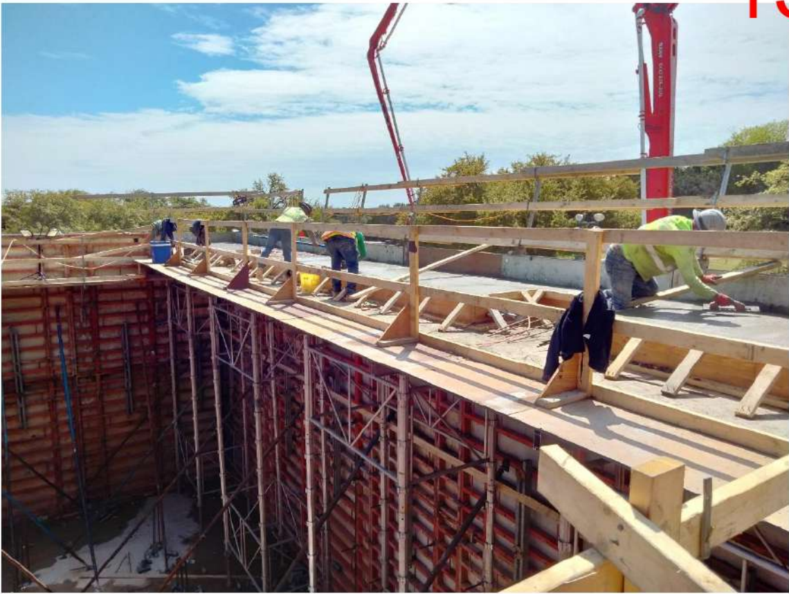
2024.03.19, Concrete Troweling Aeration Walkway
