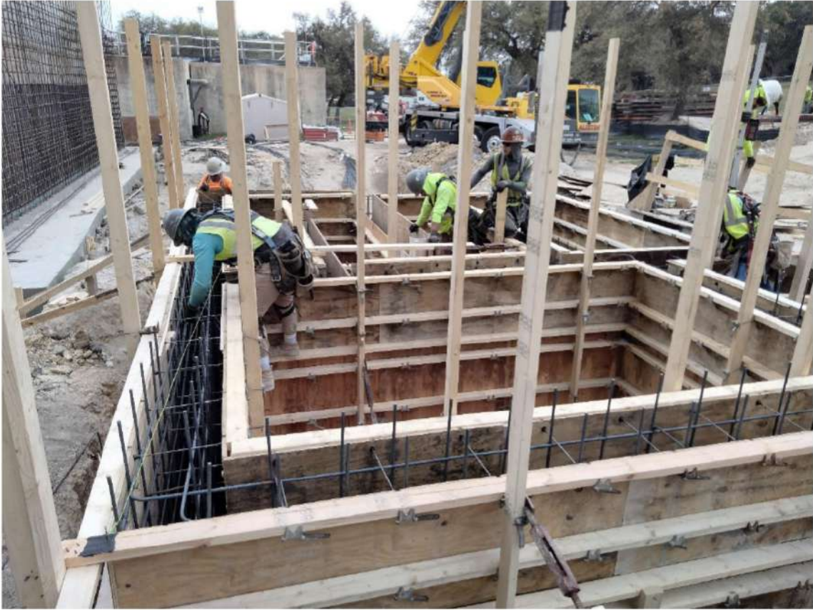
2024.03.07, CL2/Effluent Basin Rebar/Formwork Installation
