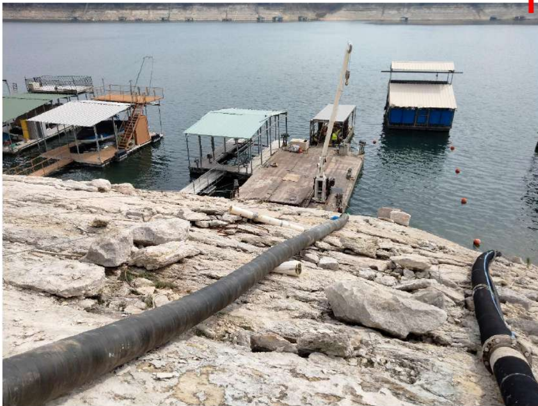
2024.02.27, Staging of Raw Water Hose
